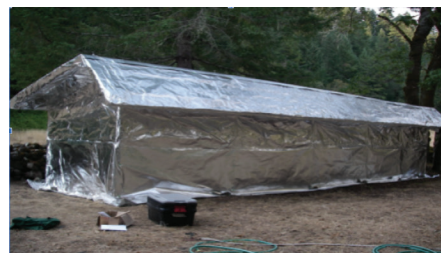
Figure 5: Black Bar Lodge. It is a structure wrapped in protective foil to prevent wildfire damage (Sonner). 20
