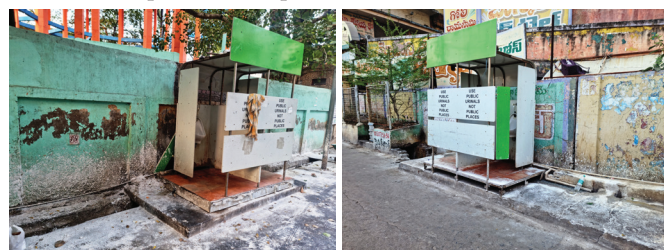
Figure 1: Unhygienic Surroundings. Figure 2: Excessive use of chemicals.
