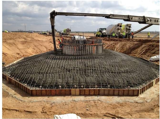
Figure 10: Example wind turbine foundation. 25 The picture shows the size of the concrete foundation used in installing a wind turbine.
