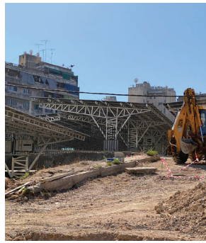
Figure 28: Site preparation for solar park. The image shows the extensive work needed for site preparation for the installation of solar panels in a solar park.
