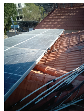
Figure 24: Wiring placement on rooftop installation. The image shows the placement of the wiring of solar panels.
