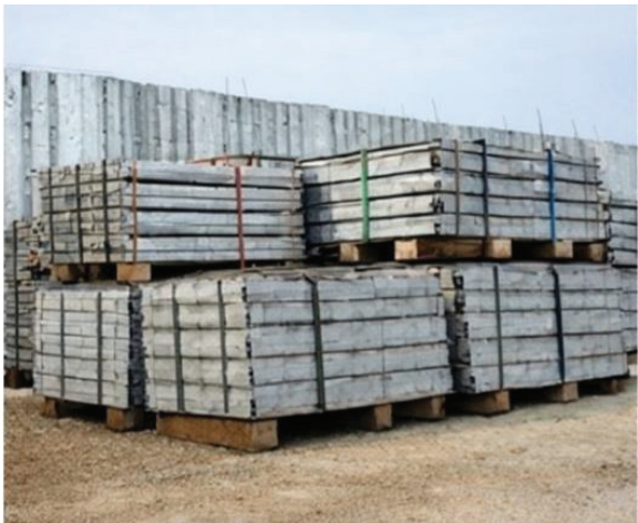
Figure 9: Proper stacking of panels for reducing contact damage and surface wear.
