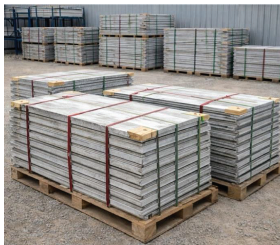
Figure 21: Correct stacking of aluminum formwork panels using protective wooden separators directly extends panel reuse life.
