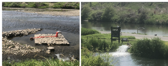
Figure 4: (1) A riverbank filtration (RBF) facility was built along the riverbed to allow for the extraction of subsurface water through infiltration and gravel-based filtration. (2) Water is being pumped from the RBF system to a nearby wetland site to improve the ecology and hydrology.
